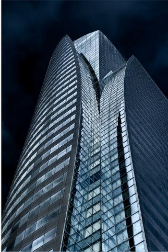
SUPERSET & GOM Bruce Barton Sathorn Square Building Bnkok
